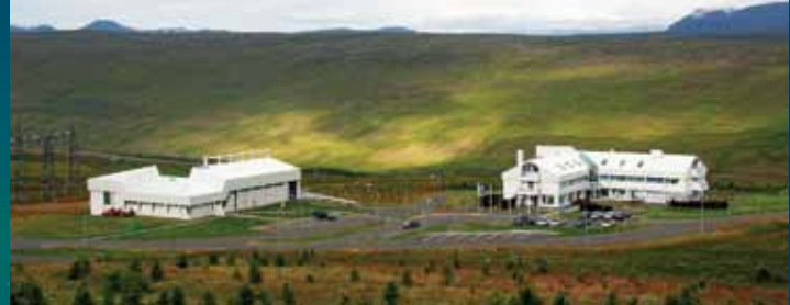
Blanda Hydropower Station located in the near Skagafjordur area – installed power capacity of 150 MW.
